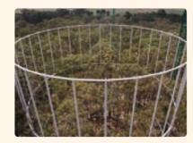
Exel Composites supplied six identical experimental 'arrays' inside the forest. Each array is served by a permanent tower crane and comprises 32 CO<sup>2</sup> vent masts 28 metres high in a 25 metre circle, surrounding a group of old-growth trees. The vent structure is fabricated from pultruded glass-fibre composite material.
