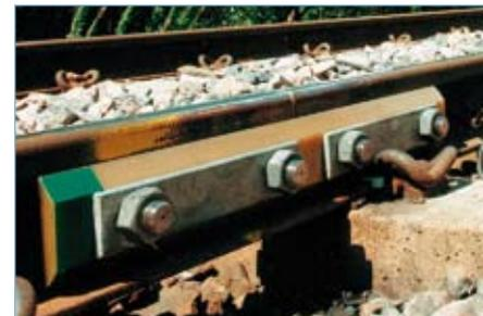
Special joints, as sample Emergency repair joints, distinctively coloured for attention. Weight per joint appr. 20 kg.
