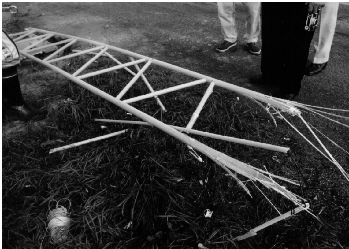
Figure A1.19 The cables and the cover tubes were cut by the impactor as can be seen.
