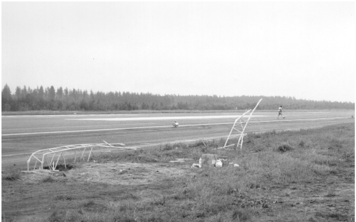
Figure A1.10 The mast broke into two main sections and into numerous separate parts.
